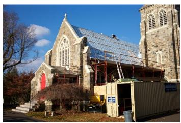
condition and needed no repair. Work continues to repair the Steeple roofing, installing new copper flashing (very flashy indeed!), and snow guard supports.
