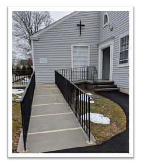
Stairs and Ramps - The front patio and stairs from the parking lot, and the stairs and ramp at the Church end of the Parish Hall, like their counterparts at the Church, were crumbling and unsafe – the result of poor drainage and original use of sub-standard materials. The front patio, stairs and the side stairs, walkway and ramp were
