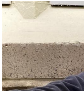
Original (1917) cast stone – cleaned section at bottom
