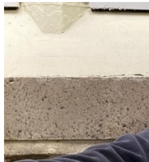
Original (1917) cast stone – cleaned section at bottom
