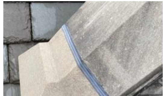
New (2015) cast stone – cleaned section at left
